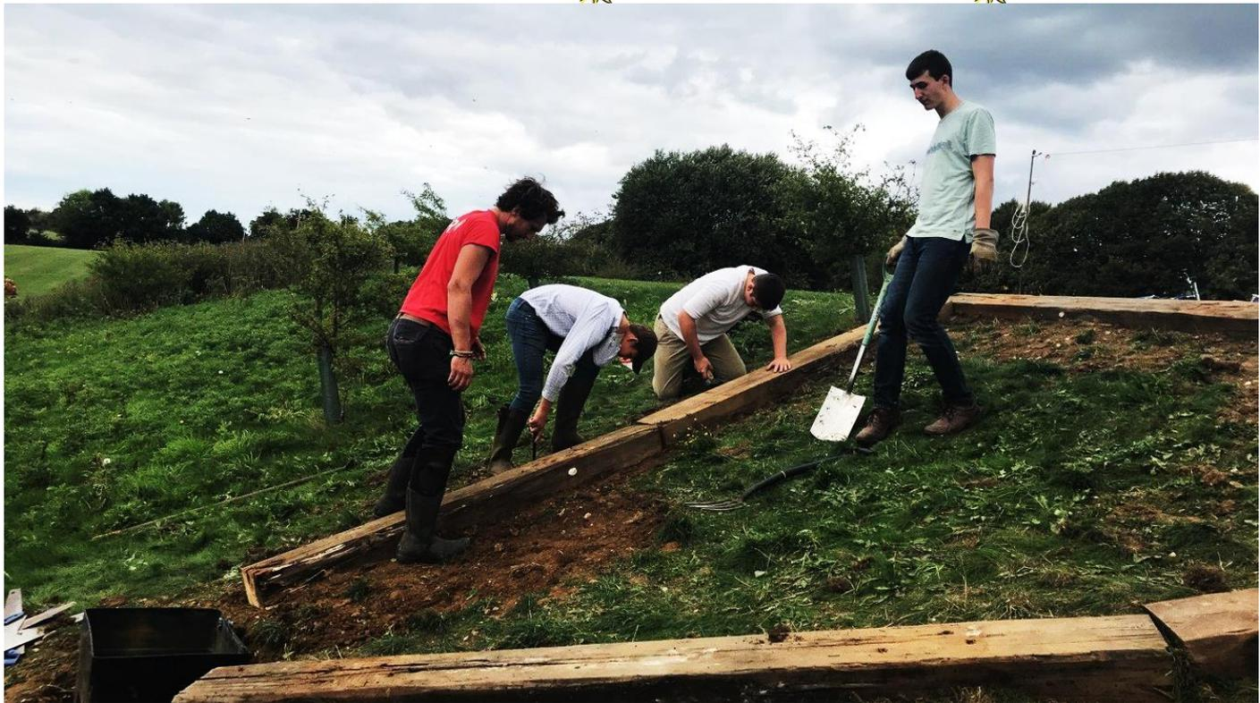
It's paramount that the sail is pinned down very firmly otherwise, being a sail, if the wind catches it, it will certainly blow away. Pinning a sail to heavy railway sleepers would be ideal. You can also attach side guttering to the railway sleepers to avoid rainwater running off the sides of the sail and not into the loft tank where you want it to go.
