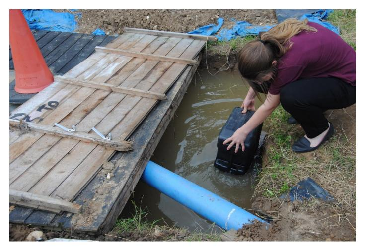
**Above:** A purpose dug water reservoir with a water pipe installed to also help collect surface water. This example was dug into heavy clay soil which naturally held the water, but a pond liner could also be used to do just the same. Notice the make shift cover to make sure than animals and people don't fall in by accident.
