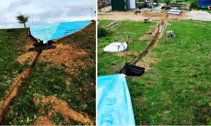
**Above:** The loft tank (the black box in images above) is merely a holding tank for the thousands of litres that a sail catcher can collect. Thinking sensibly about water storage and where all this water goes is essential. Please read the storage section of this article for ideas about this along with the health and safety behind storing water too.
