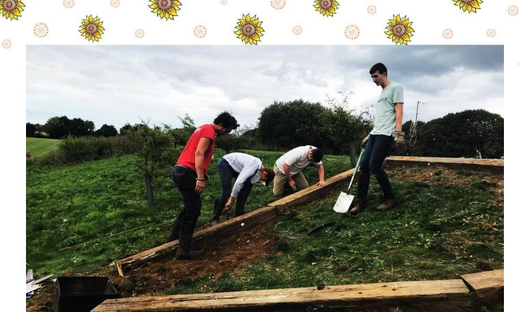
It's paramount that the sail is pinned down very firmly otherwise, being a sail, if the wind catches it, it will certainly blow away. Pinning a sail to heavy railway sleepers would be ideal. You can also attach side guttering to the railway sleepers to avoid rainwater running off the sides of the sail and not into the loft tank where you want it to go.
