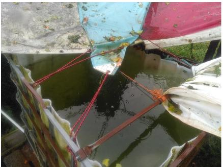
Left: The tops of IBC tanks can also be removed to collect more rainwater like a water butt does. Although the metal cage does continue to provide structure, it does mean that, with the lid off, there is more of risk of leaves, animals and people falling. The example opposite shows how old sails, fixed and aimed downwards towards the IBC, are incredibly effective at collecting rainwater.
